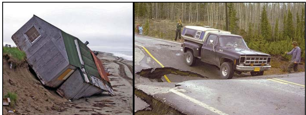
Figure 9.12: Melting permafrost has caused a house in Shishmaref, Alaska to topple; on the Alaska Highway, permafrost subsidence caused the road to collapse under the weight of a pickup truck.
