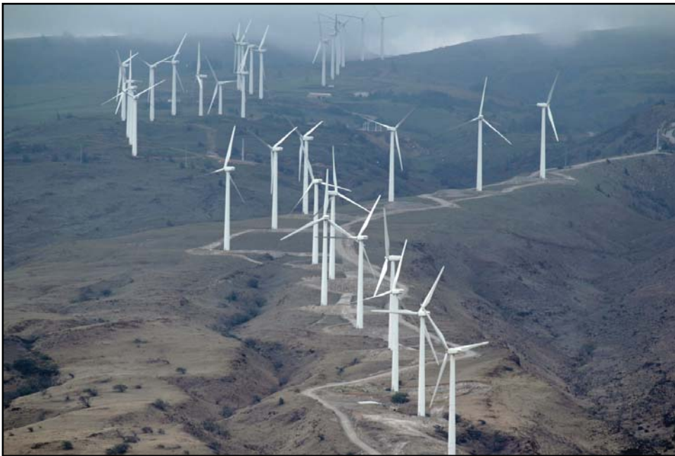
Figure 7.6: Kaheawa Wind Farm, Maui.
