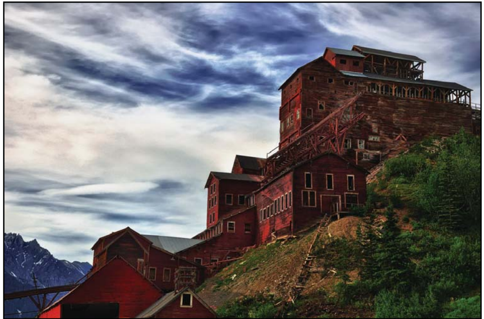
Figure 5.18: The 14-story concentration mill at the Kennicott Copper Mine, built in 1906. Today, the mill and mines are located in Wrangell-St. Elias National Park & Preserve.
