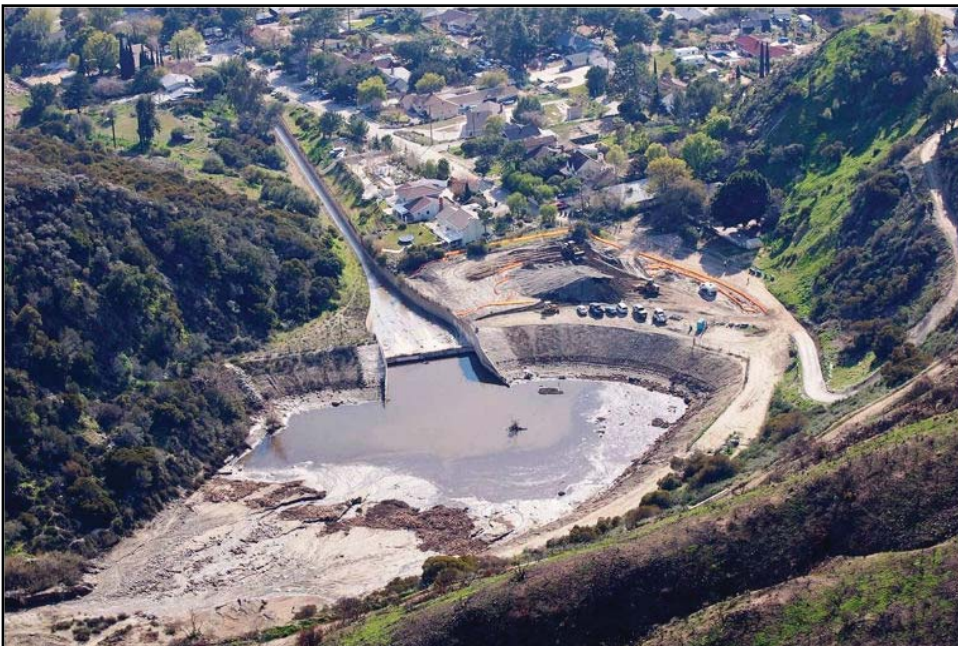
Figure 10.13: This debris basin in Los Angeles county is designed to capture the sediment, boulders, and other debris washed from the canyon during a storm.
