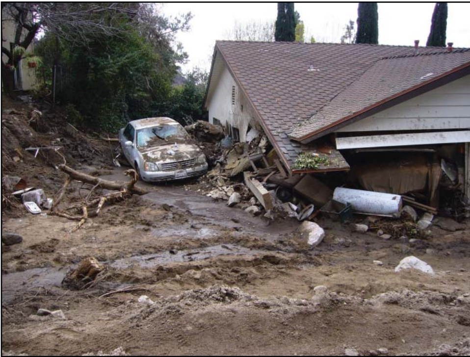
Figure 10.12: This debris flow occurred on February 6, 2010 in La Canada-Flintridge, California as a result of a flash flood generated in Mullally Canyon.
