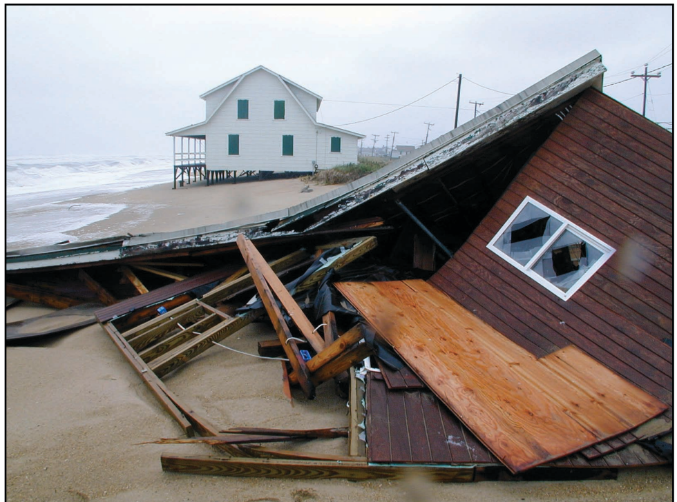
Figure 9.26: A beach house is undermined and destroyed by storm surge from Hurricane Dennis in 1999, at Kitty Hawk, North Carolina.
