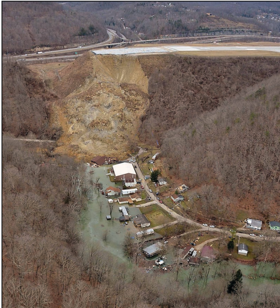
Figure 9.9: The landslide below Yeager Airport in Charleston, West Virginia damaged houses, blocked a creek, and covered a road.
