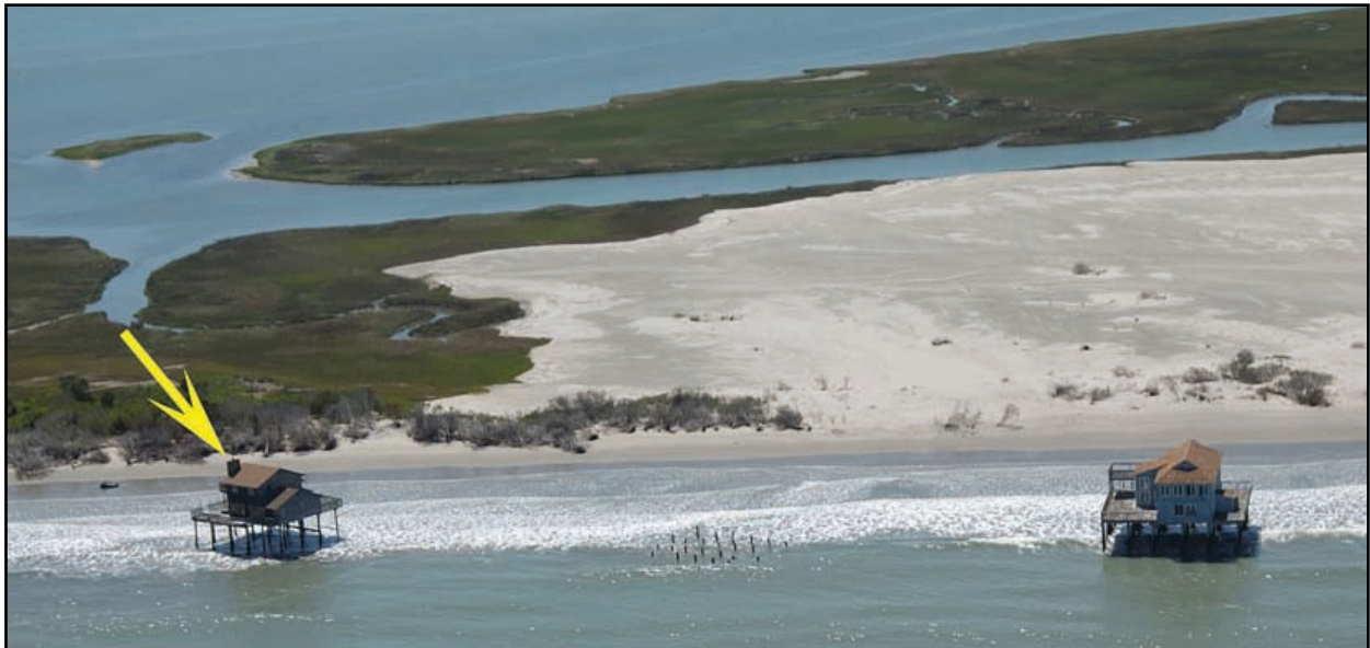
Figure 9.27: These houses on Cedar Island, a barrier island off Virginia's coastline, were originally built on solid ground. As sand on the island migrated, the buildings were left behind (shown by the yellow arrow).
