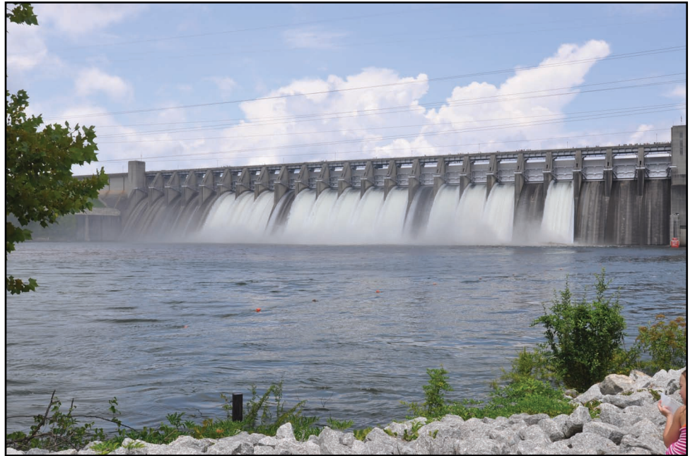
Figure 6.8: The J. Strom Thurmond Dam (also known as Clarks Hill Dam) is located on the Savannah River at the border of Georgia and South Carolina. The 334-meter-wide (1096-foot-wide) dam houses a 380 MW hydroelectric plant.
