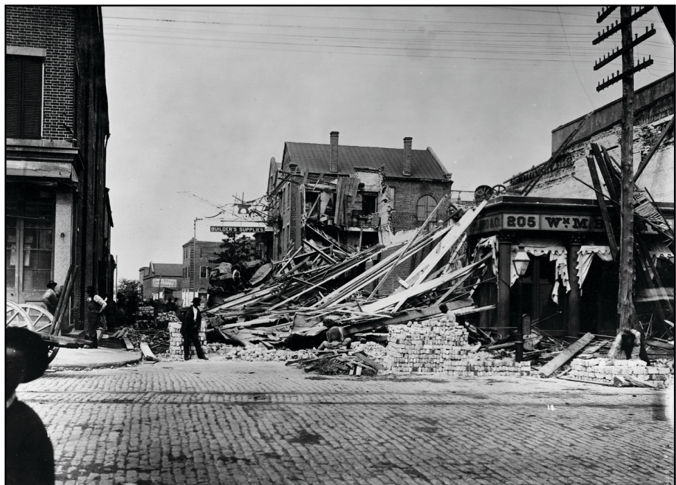
Figure 9.4: Rubble and collapsed buildings line the streets of Charleston, South Carolina, after the devastating 1886 earthquake.
