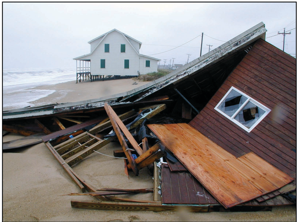
Figure 9.26: A beach house is undermined and destroyed by storm surge from Hurricane Dennis in 1999, at Kitty Hawk, North Carolina.
