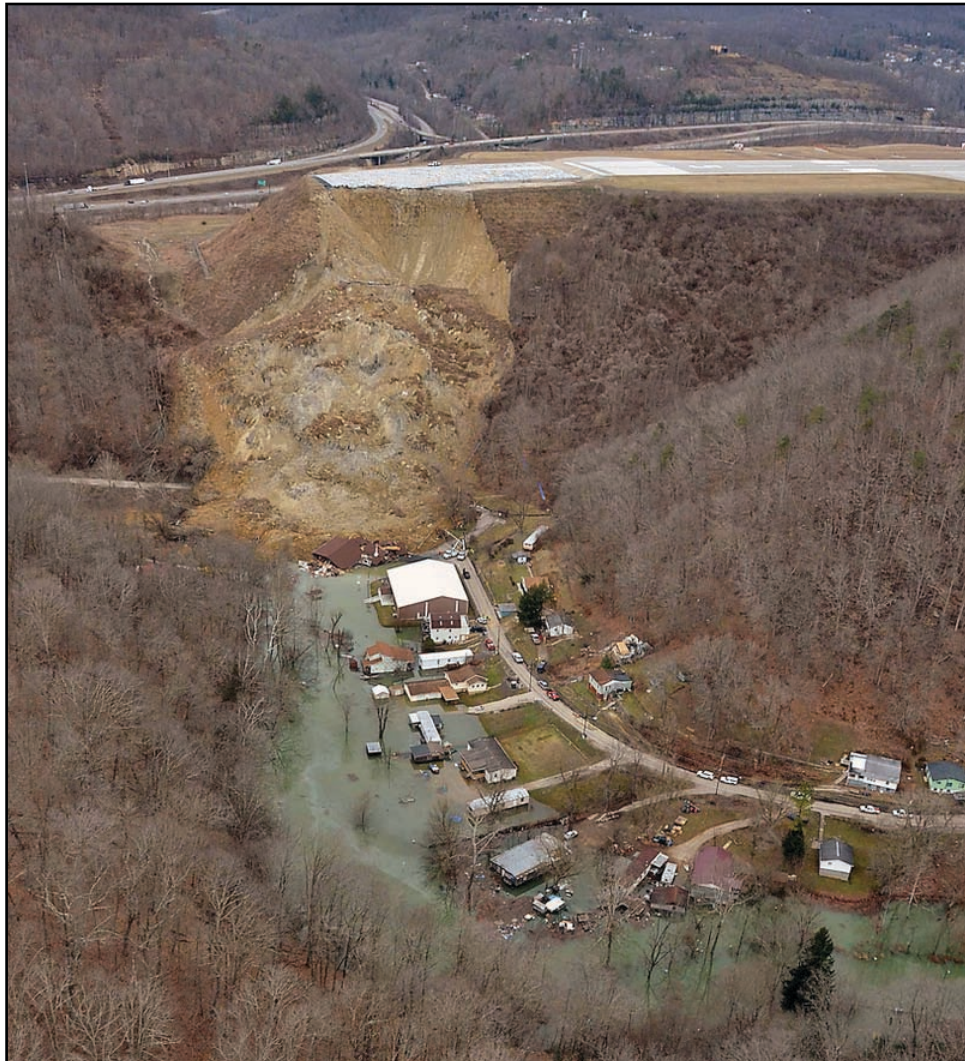
Figure 9.9: The landslide below Yeager Airport in Charleston, West Virginia damaged houses, blocked a creek, and covered a road.
