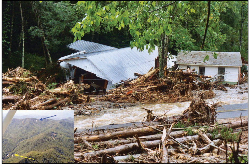
Figure 9.10: A pile of trees, debris, and homes detached from their foundations after the Peeks Creek landslide in Franklin, North Carolina. Inset shows the track of the landslide, from the start (blue arrow) to the Peeks Creek community (yellow arrow). (See TFG website for full-color version.)
