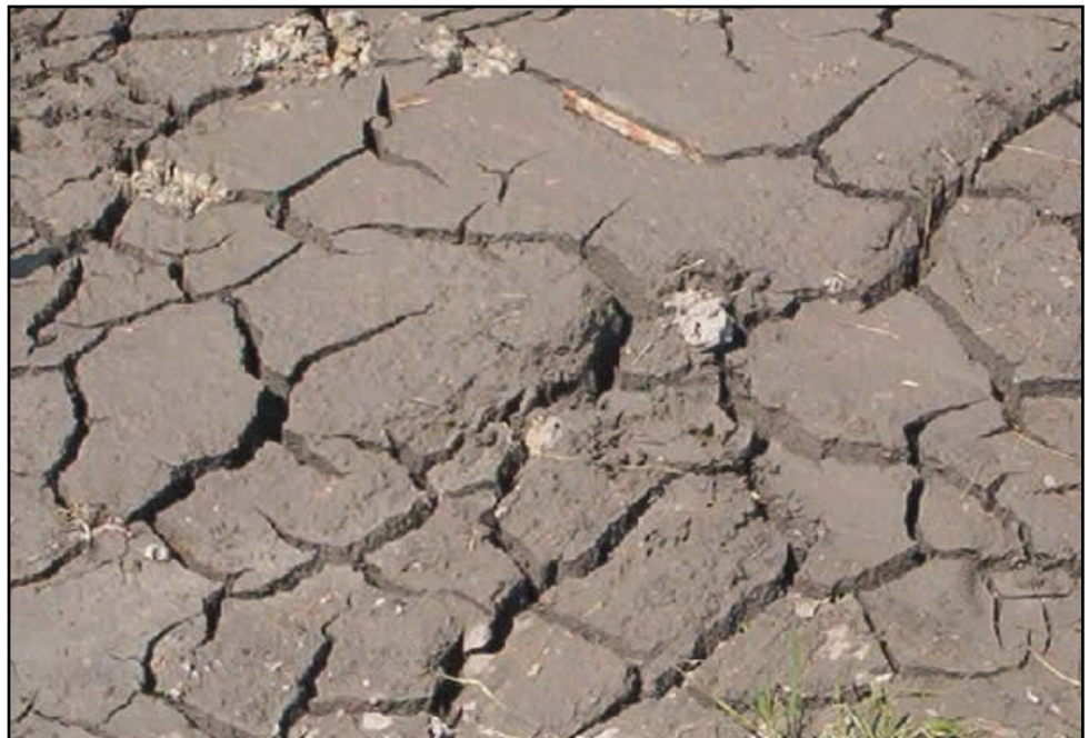
Figure 7.24: Cracked Vertisols near Birmingham, Alabama.
