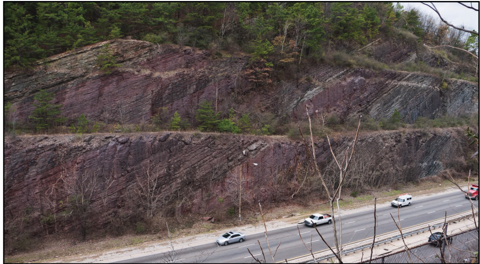
Figure 2.26: The Silurian sandstone strata of Red Mountain are exposed along this roadcut on the Red Mountain Expressway, near Birmingham, Alabama.
