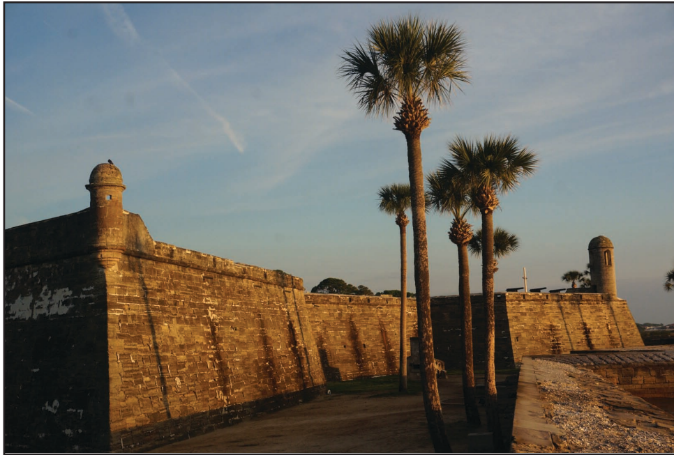
Figure 2.38: The Castillo de San Marcos, a 17th century fort in St. Augustine, Florida, was constructed from coquina.
