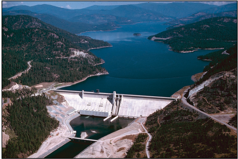
Figure 7.14: Libby Dam, on the Kootenai River in Lincoln County, Montana. This dam is 129 meters (422 feet) tall and 931 meters (3055 feet) long, with a generating capacity of up to 600 megawatts.
