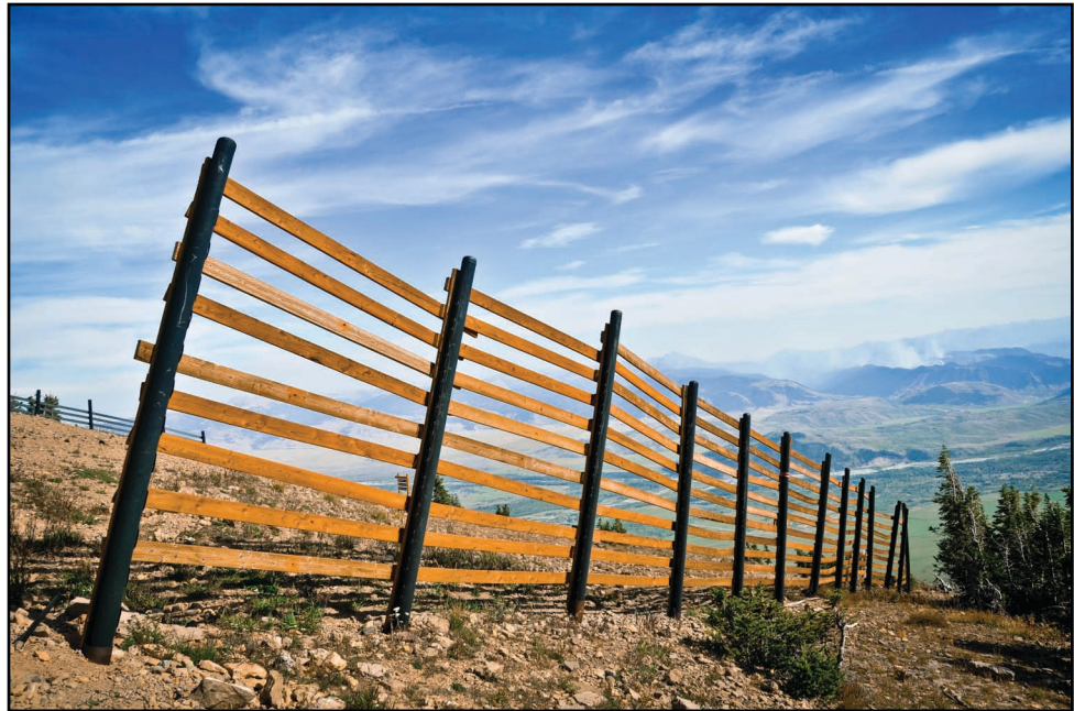
Figure 9.11: A snow fence near the Grand Tetons in Wyoming. Fences like these are used to force windblown snow to accumulate in a desired place, keeping it off roadways or collecting it for later use as a water supply.
