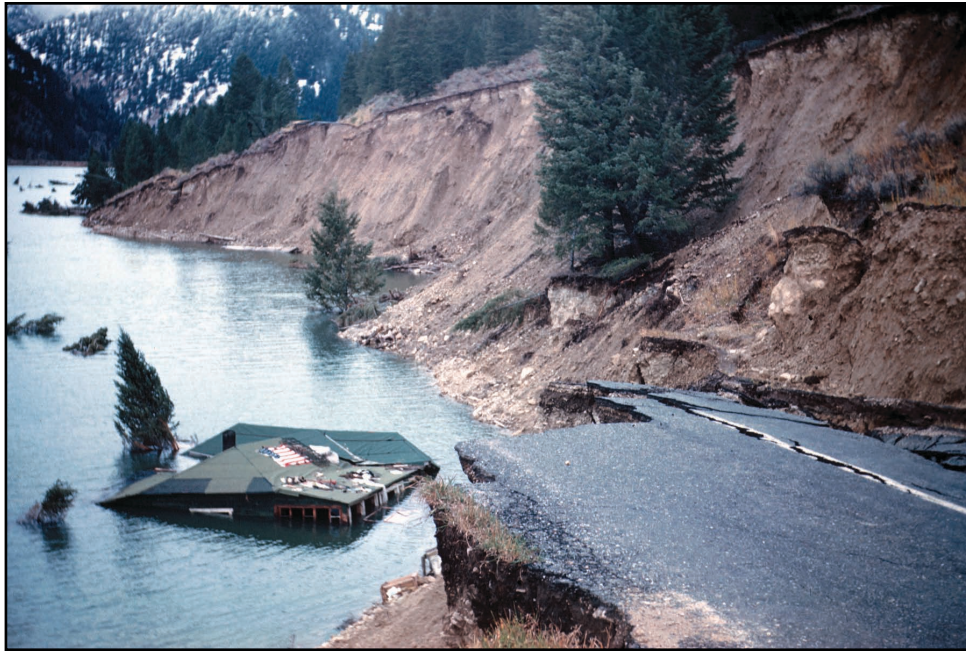
Figure 10.6: Earthquake damage to State Highway 287 and the Hilgard Lodge near Hebgen Lake, Montana.
