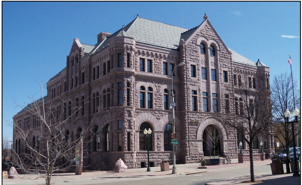
Figure 2.3: Sioux Quartzite was used to construct the Federal Building in Sioux Falls, South Dakota.
