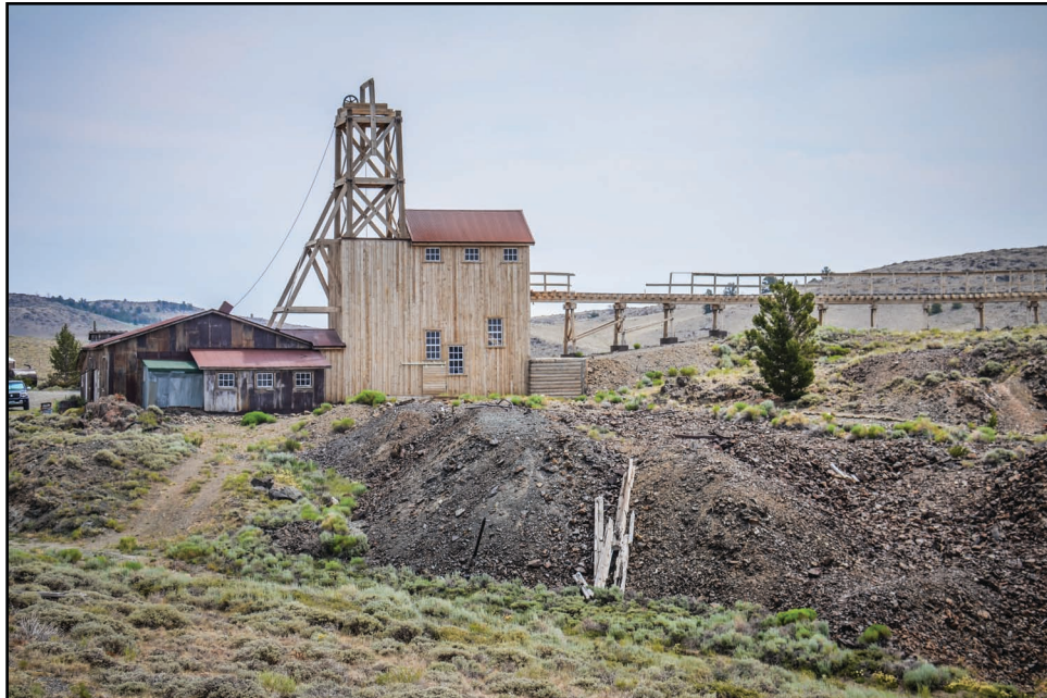
Figure 5.19: The Carissa Gold Mine, which operated from 1867 to 1954. In 2003, the state of Wyoming restored the mine and mill as a historic attraction.
