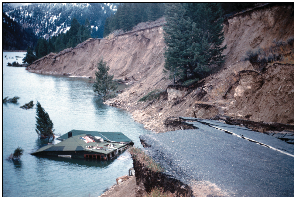
Figure 10.6: Earthquake damage to State Highway 287 and the Hilgard Lodge near Hebgen Lake, Montana.
