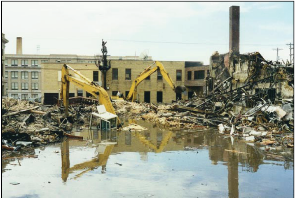
Figure 10.26: Wreckage in Grand Forks, North Dakota, after the 1997 Red River Flood.
